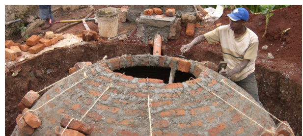
One of the first biogas units just before completion. At the moment more than a dozen specialised masons are doing the construction work of the installations.
